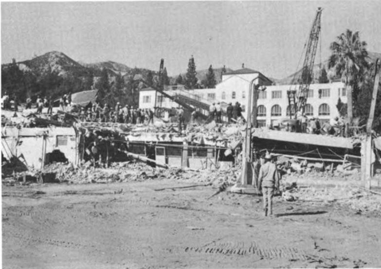
**FIGURE 4** Collapsed portion of Sylmar Veterans Hospital being removed in search for survivors. The last of 14 survivors was found shortly after this photograph was taken. In this Hospital, built before the current building codes were established, 42 people were killed. *Photograph courtesy of Earthquake Engineering Research Laboratory, California Institute of Technology.*
