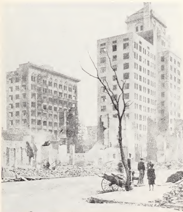
FIG. 17. Augusta, Georgia Fire, 1916. Fire resistive buildings with ordinary glass windows were gutted, along with 680 other buildings.
