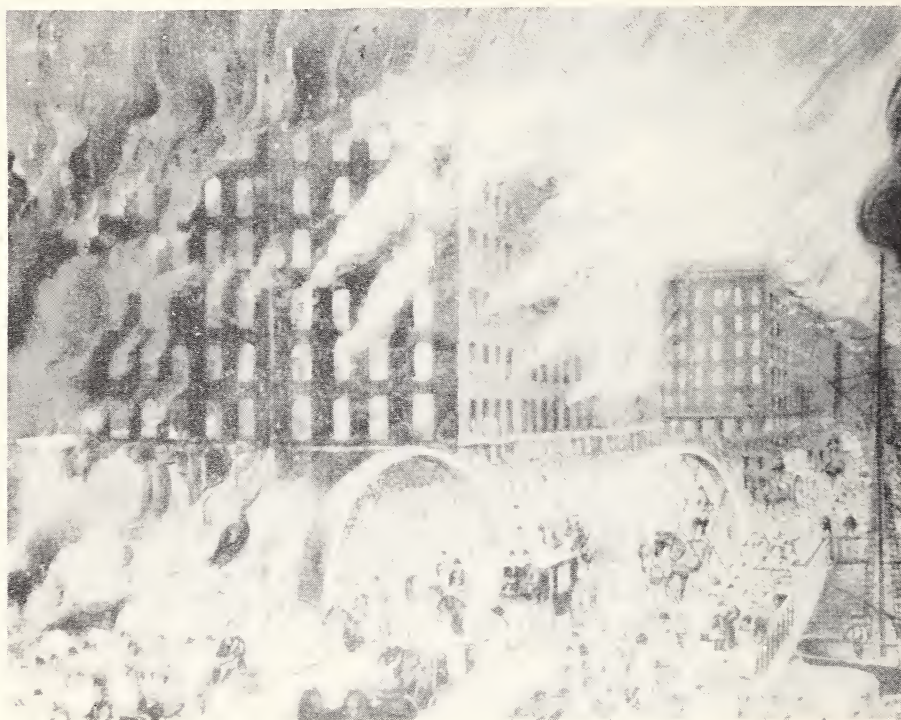
FIG. 1. Currier & Ives of State Street Bridge.
