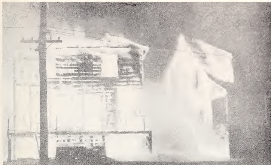
FIG. 14. Fire spreading from house to house, far beyond the range of licking flames; Hull, Massachusetts, 1923.
