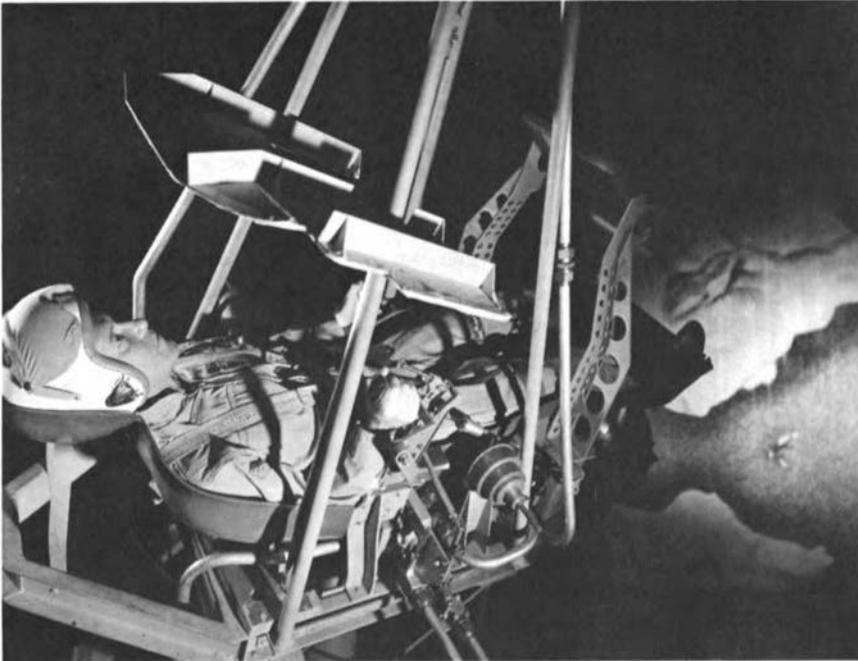
Figure 2. MB-3 simulator: a second stage of fixed-base attitude control simulation which incorporated the astronaut's couch, pressure suit, and Mercury hand controller.
