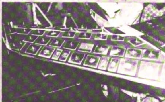
HIMAT WING WITH LOAD PADS
