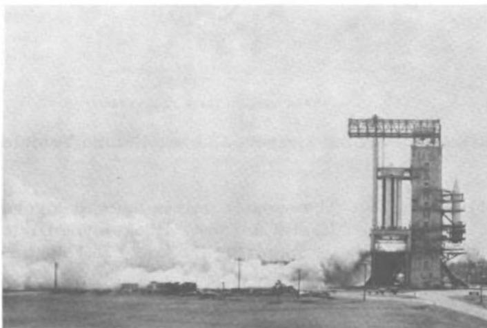
Figure 65. SATURN Booster During Static Firing
