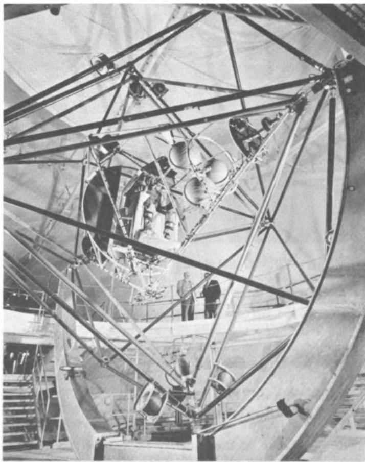
Figure 74. The Multi-Axis Test Facility installed in the altitude wind tunnel. A pilot is shown in the support couch.
