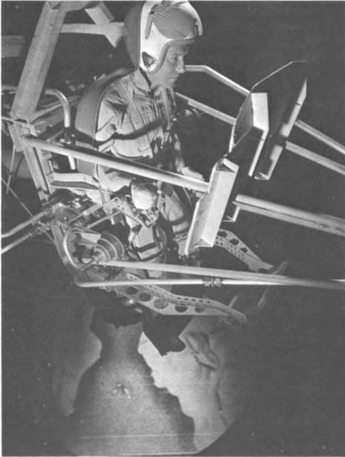
**Figure 73. Orbital Air Bearing Simulator**
