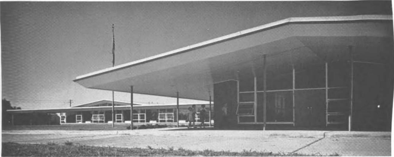
**Fig. 4.33—Small and large glass areas used together with ample overhang to provide sun and rain protection, Elementary School, Port Arthur, Tex.**
