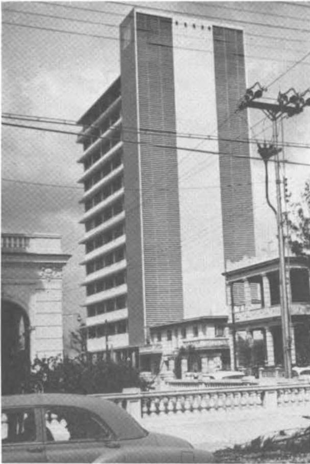
Fig. 1.26—Horizontal louvers set out on the western exposure; balconies on the southern exposure of an office building in Havana, Cuba.
