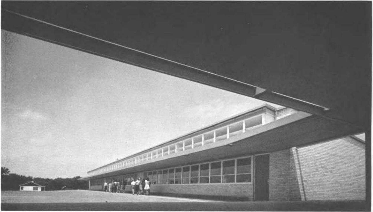
**Fig. 4.31**—Low glass area used for visual aid and light, protected by overhang; high glass area used for light only with interior horizontal sun control louvers, Westwood Elementary School, Stillwater, Okla.
