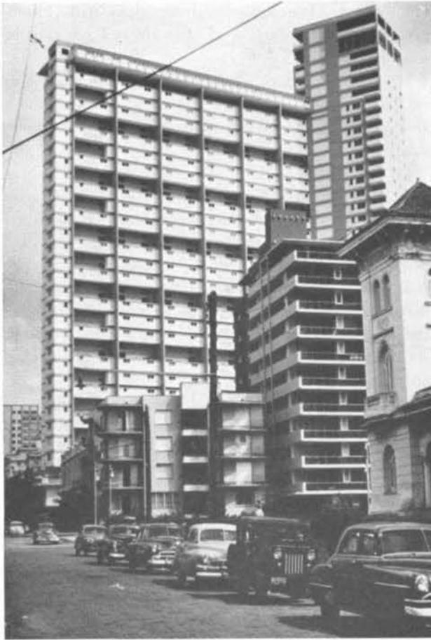
Fig. 1.24—Overhanging balconies, etc., on the southeastern exposure of an apartment house in Havana, Cuba.
