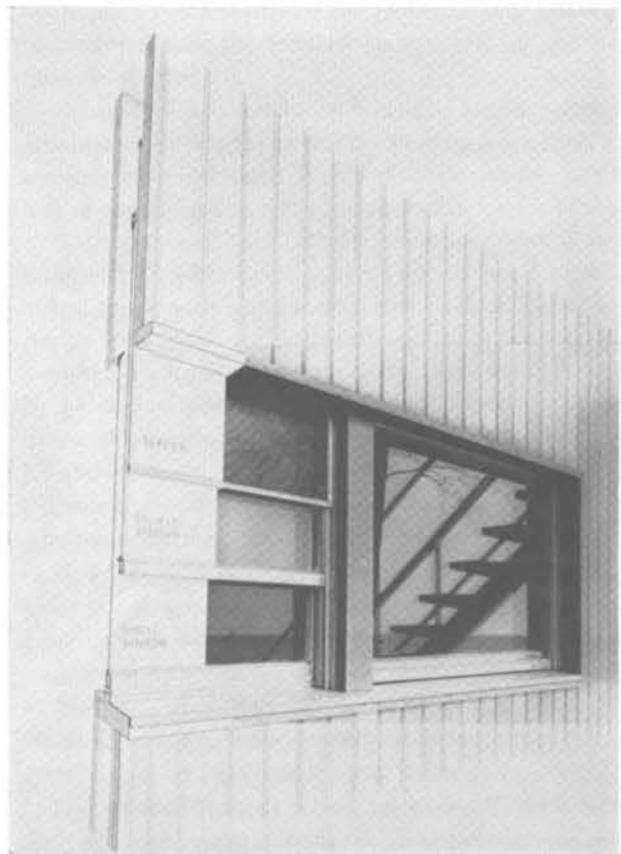
Fig. 4.2—Aluminum window designed by George Fred Keck and manufactured by Adams and Westlake, as installed in 1940 in a residence in Menasha, Wisconsin.
