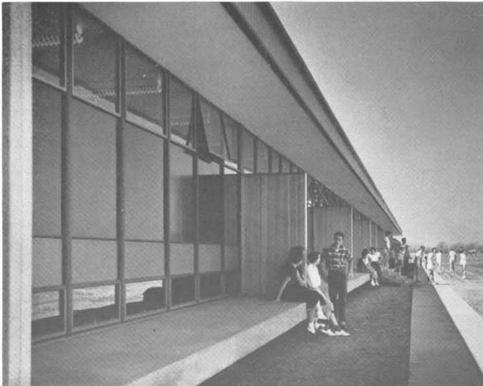
**Fig. 4.32**—Combination of clear and glare-reducing glass with roof overhang, Norman High School, Norman, Okla.
