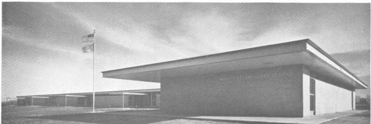
Fig. 4.30—Use of high brick walls on north and west with small glass area for light distribution, Madison Elementary School, Norman, Okla.
