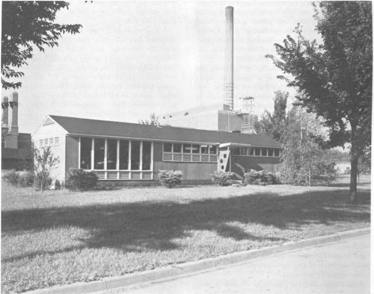
Fig. 4.4—Small Homes Council Laboratory showing windows on north elevation with ventilating units underneath fixed glass.
