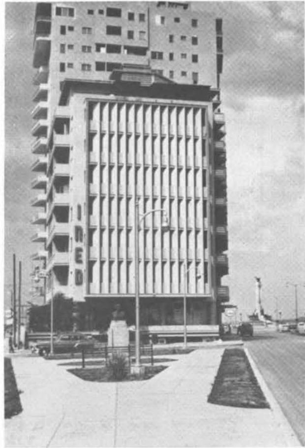
Fig. 1.27—Vertical concrete included louvers on the western exposure of an apartment house in Havana, Cuba.
