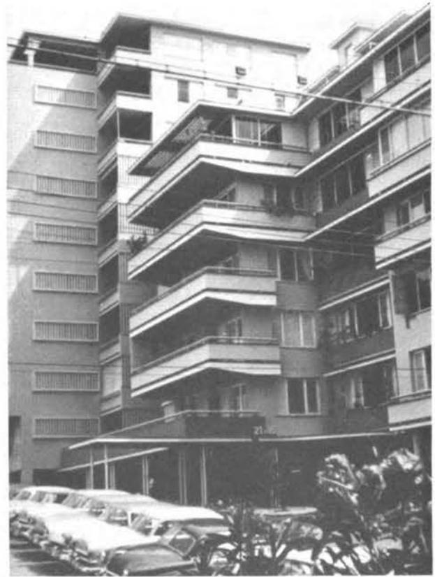
Fig. 1.25—Projecting balconies to southeast and louvers to the northeast in an office building in Havana, Cuba.
